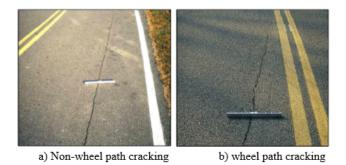
Figure 3: Longitudinal cracking on the pavement surface
