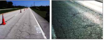
Block cracking on the pavement surface
