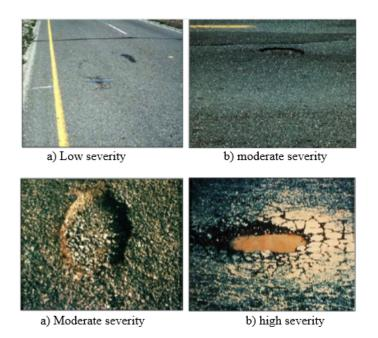
Figure 4: Potholes on the pavement surface
