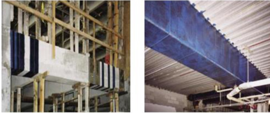
Figure 2: FRP flexural and shear reinforcement
