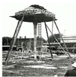
Figure (5). Testing the columns for the Johnson Wax Building, Frank Lloyd Wright, 1936 [5]
