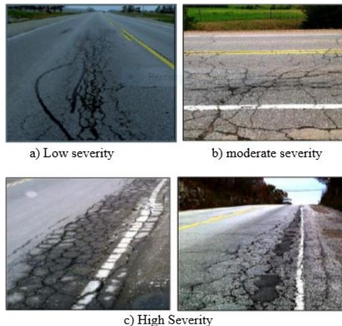
Figure 1: Sample Fatigue cracking on the pavement surface a) low severity b) moderate severity c) high severity
