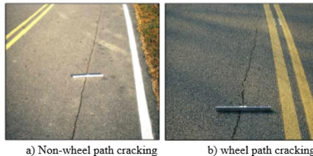
Figure 3: Longitudinal cracking on the pavement surface
