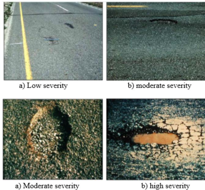
Figure 4: Potholes on the pavement surface
