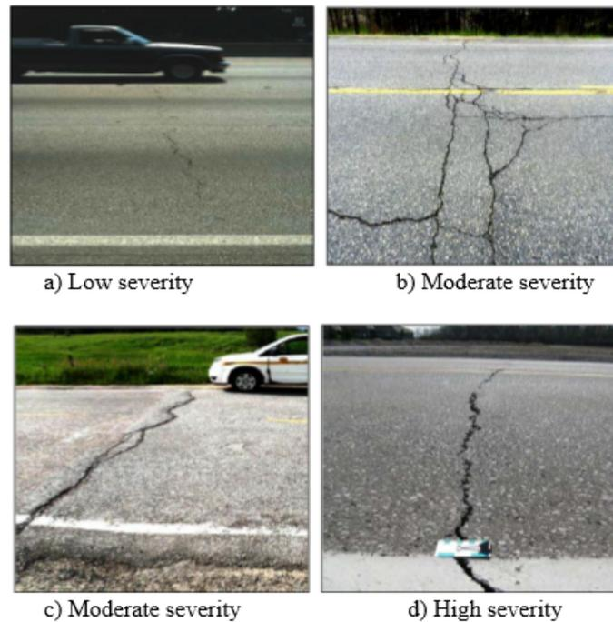
Figure 2: Transverse cracking on the pavement surface showing a) low severity b) and c) moderate severity d) high severity
