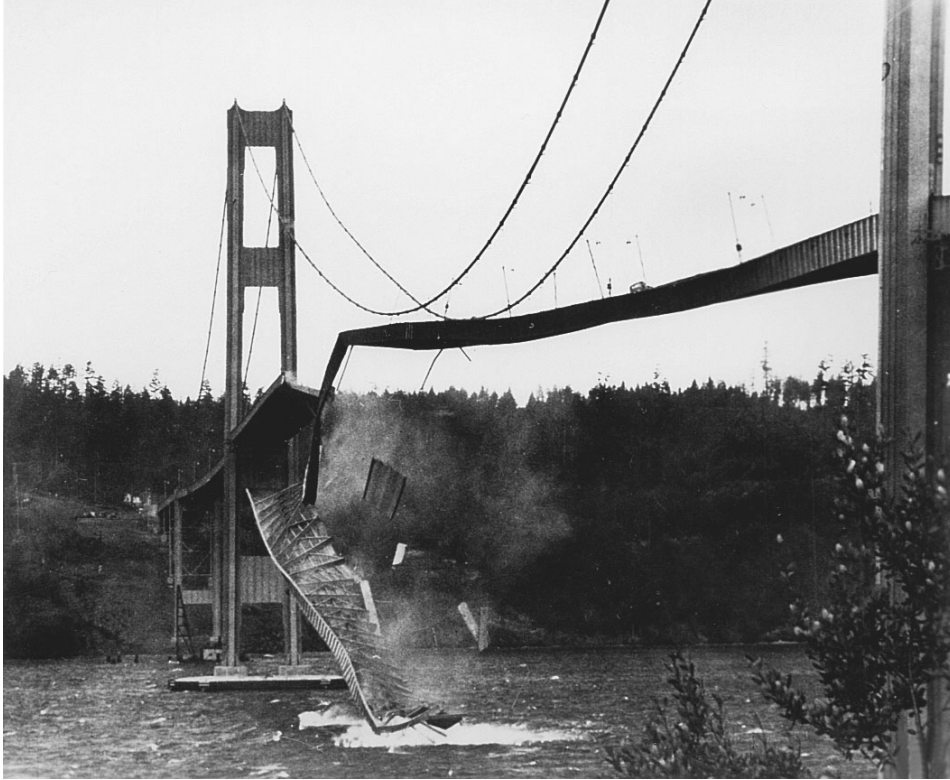
Figure 1: Collapse of the Tacoma Narrows Bridge.
